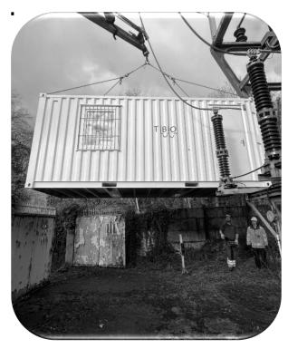
Unloading an ODB System® installation, pre-assembled in a 20' maritime container
